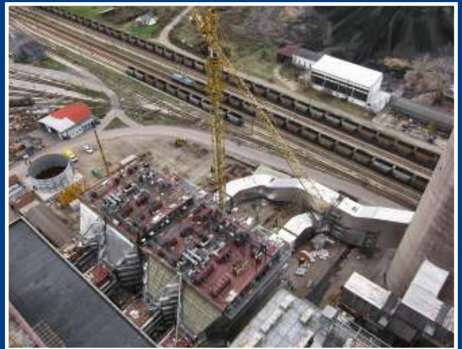
Erection of Unit A6 ESP in Obrenovac
