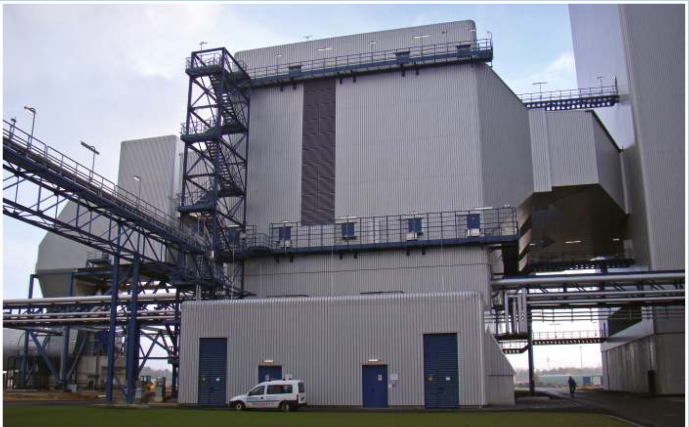
Boxberg Unit no. R – 670 MW – manufacturing, delivery, erection and commissioning
